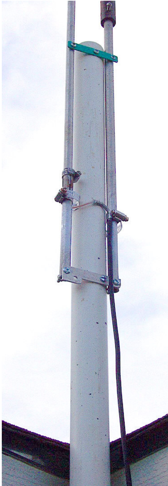
Notice the hollow insulator covering the air gap at the top of picture.
